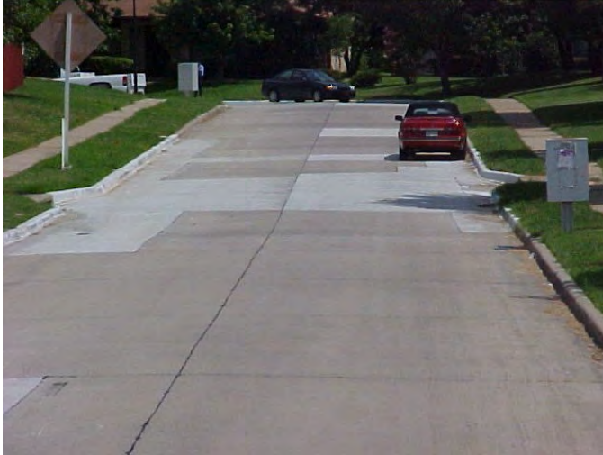
Subdivision Street After Patching And Slab Repair.
