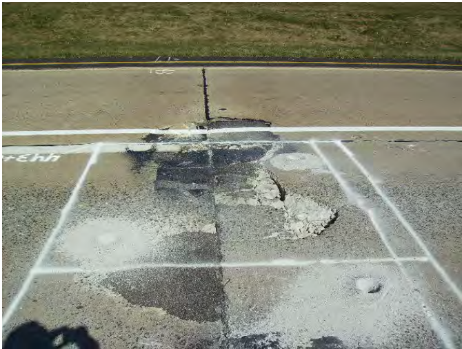
Failed Section Marked For Replacement
