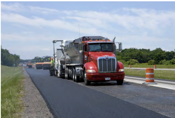
Overlay Paving Operation
