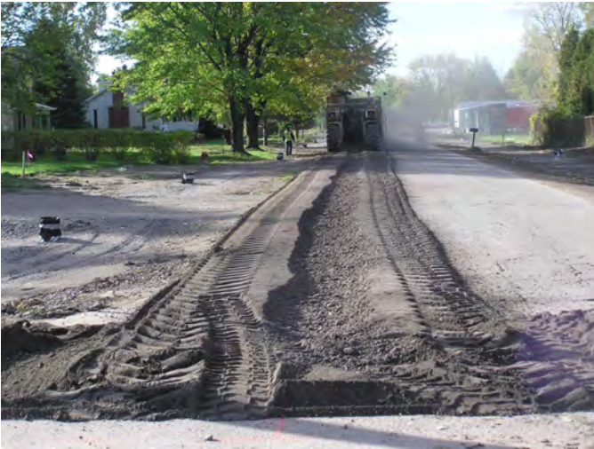
Pulverizing Existing Pavement Prior To Overlay
