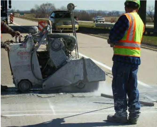
Saw Cutting Section For Removal
