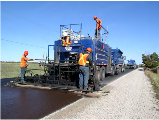
Slurry Seal Application
